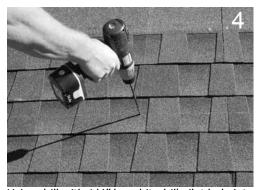
roof and rafter, taking care to drill square to the ant. roof. Do not use Mount as a drill guide.
