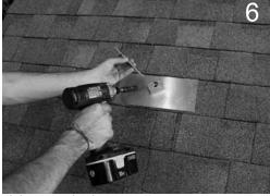
Using drill with 1/4" long bit, drill pilot hole into Clean off any saw dust, and fill hole with Seal- Slide Mount back into position. Prepare Hanger Bolt with 1 Hex Nut and 1 Sealing Washer, insert through Block into hole and drive Hanger Bolt into rafter, tightening to 13 foot Pounds.
